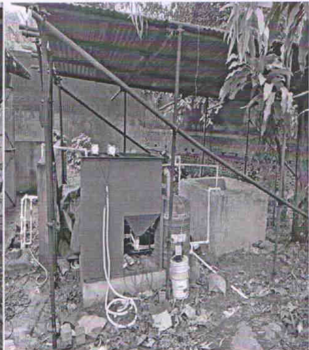
Picture – 4 (Sinter Plant)
